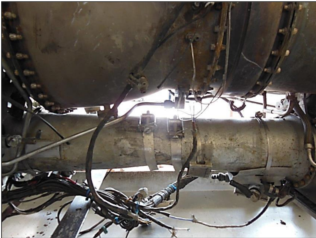
The link tube caved in at rear support level
